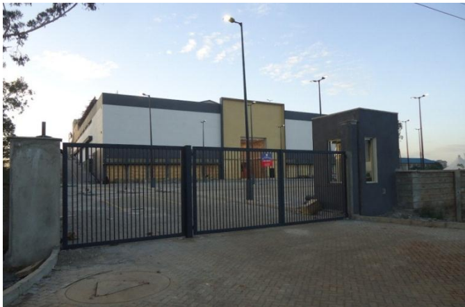
Fig 4.49: Thika Road Mall front entrance at completion, showing steel gate. Source; www.skyscrapercity.com Accessed 12/12/2013
