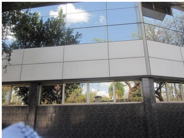
Fig 4.07: Wall tiling and glass cover the facades of the Sarit Centre. Source; Author, 2013
