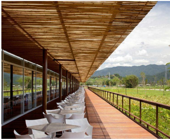
Fig 4.66: Glass, bamboo louvers and wood are materials used at Serramar. The glass gives a good view to the mountains in the distance. Source; Helm, 2012
