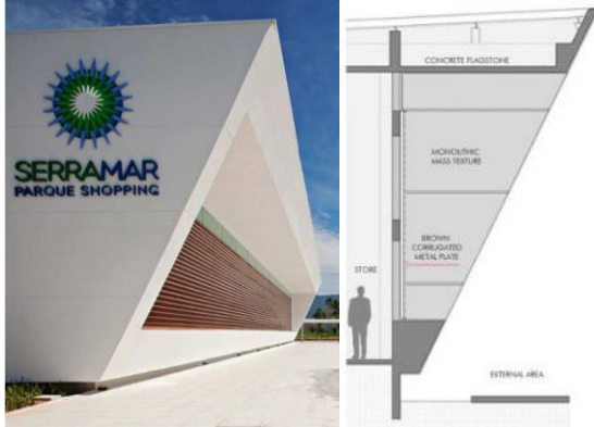
Fig 4.63: Sun-shading at Serramar Parque Shopping. Source; Helm, 2012
