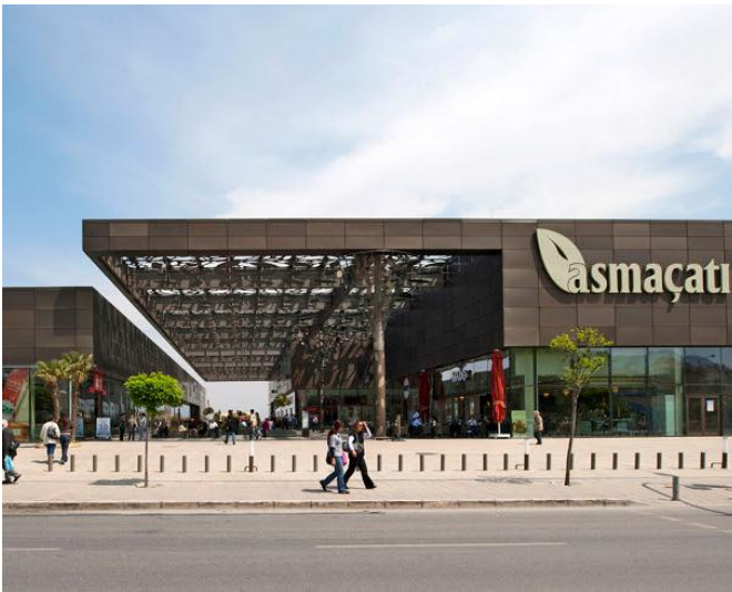
Fig 4.85: Main access corridor at Asmacati Shopping Centre. Source; Mayer, 2011
