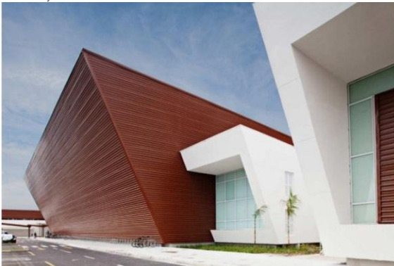
Fig 4.64: Simple finish of the blocks with a textured monolithic mass and a brown metal plate. Source; Helm, 2012
