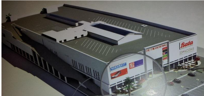
Fig 4.60: Model showing the layout of the roof-top parking with the ramp access to the extreme left façade. Source; Studio Infinity Architects
