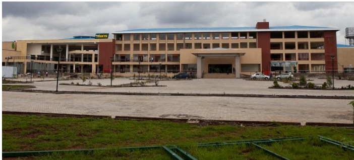
Fig 1.02: Greenspan Mall in Greenspan Estate, Umoja, Nairobi. Source; http://metrix.co.ke/html/greenspan.html . (Accessed 06/06/2013)
