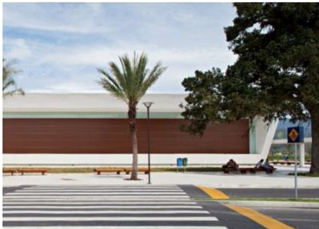
Fig 4.78: The use of road signs at Serramar Parque Shopping parking. Source; Helm, 2012
