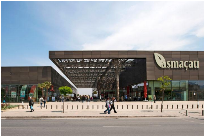
Fig 4.79: Entrance into Asmacati Shopping Centre. Source; Mayer, 2011
