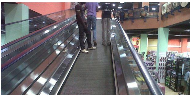
Fig 5.07: Escalating ramps at Thika Road Mall. Source; Author, 2013
