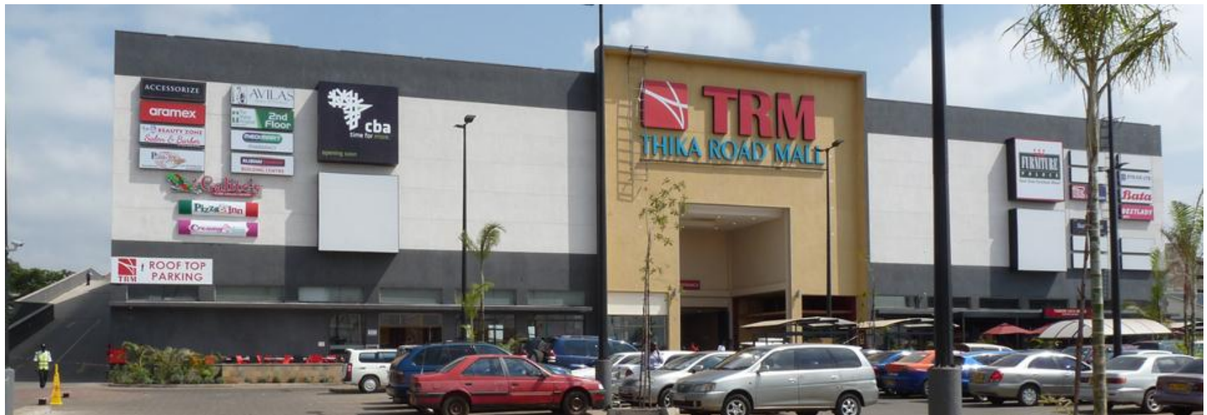
Fig 4.59: Thika Road Mall front parking showing articulation with palm trees and the ramp to the roof top parking together with the signage of the same to the far left of the image. Source; Author, 2013
