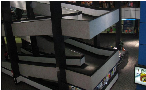
Fig 5.06: The ramps inside The Sarit Centre aid in vertical circulation of not only goods and patrons but also the disabled. Source; Author, 2013
